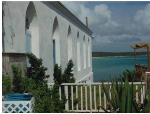
Restored colonial building in Cupids Cay overlooking Governors Harbor. Photo by Scott Gillilan.
